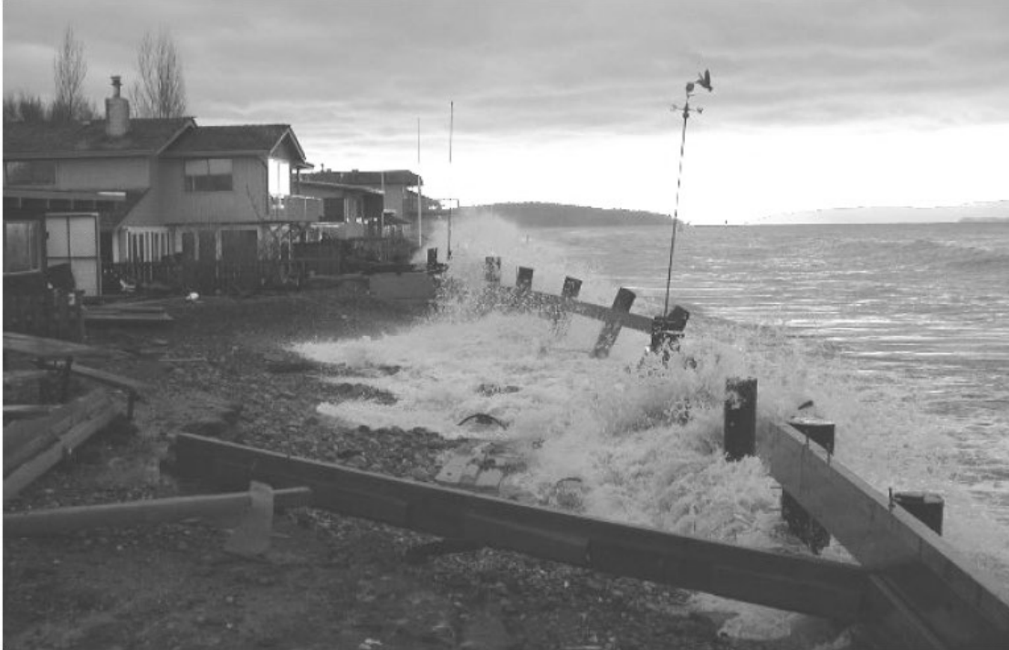
Figure 2-3 Wave Overtopping Along Sandy Point During December 2000 Storm
